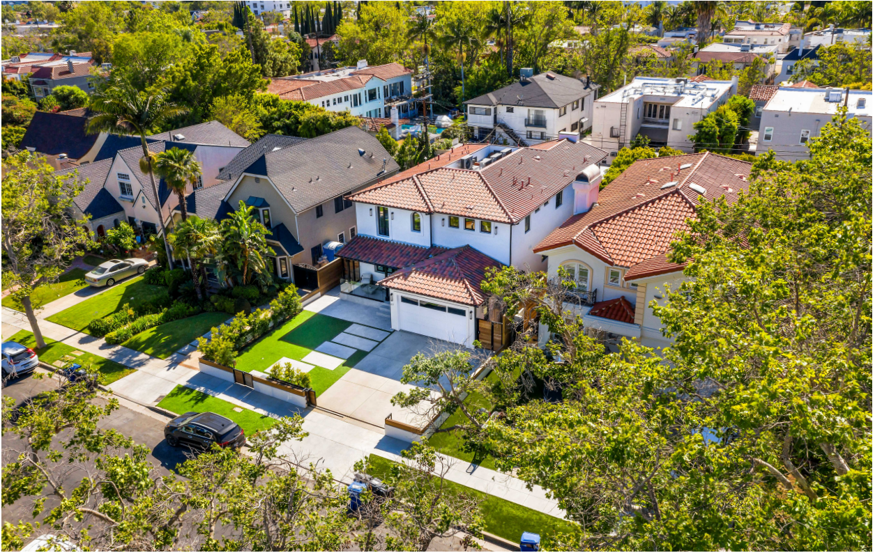
117 N Citrus Ave — Aerial View
